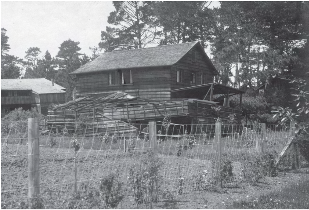
Emma Shafter Howard's house on the Inverness Mesa, seen shortly after it was damaged by the 1906 earthquake. It was later destroyed by fire and rebuilt in a different style.
